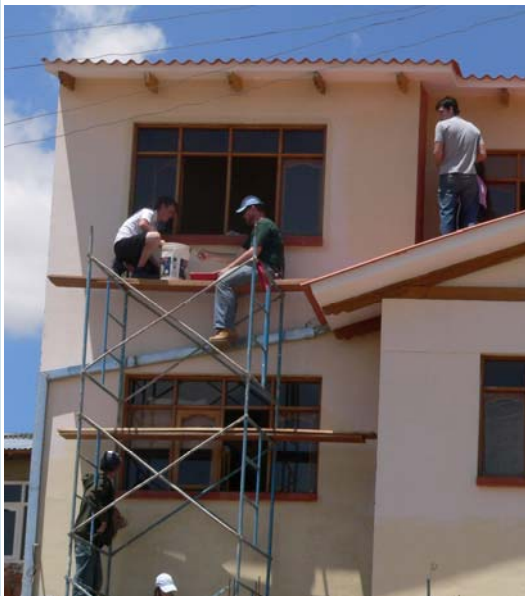
Brandon up on a scaffolding, supervising (in the middle).
